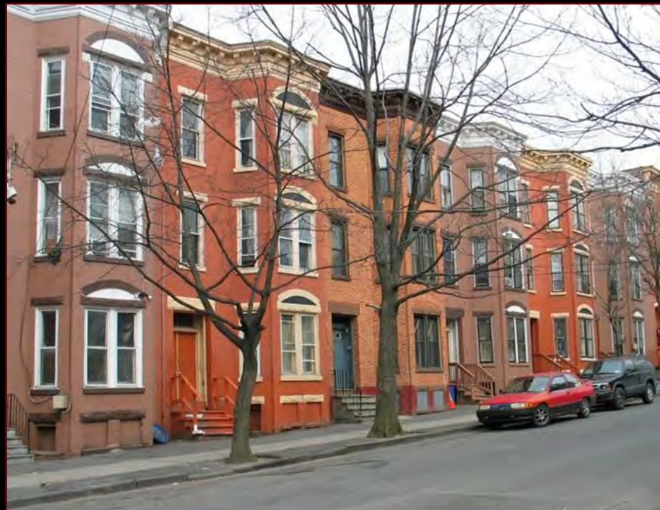
Knox Street Apartments, Albany Rehabilitation of apartments in 18 townhouses
